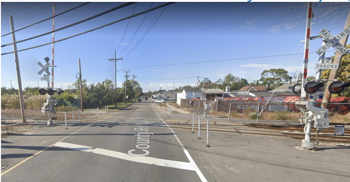
Figure 14. ROW Incursion Treatments Installed at the LIRR Crossing on 5th Ave in Bay Shore, NY
