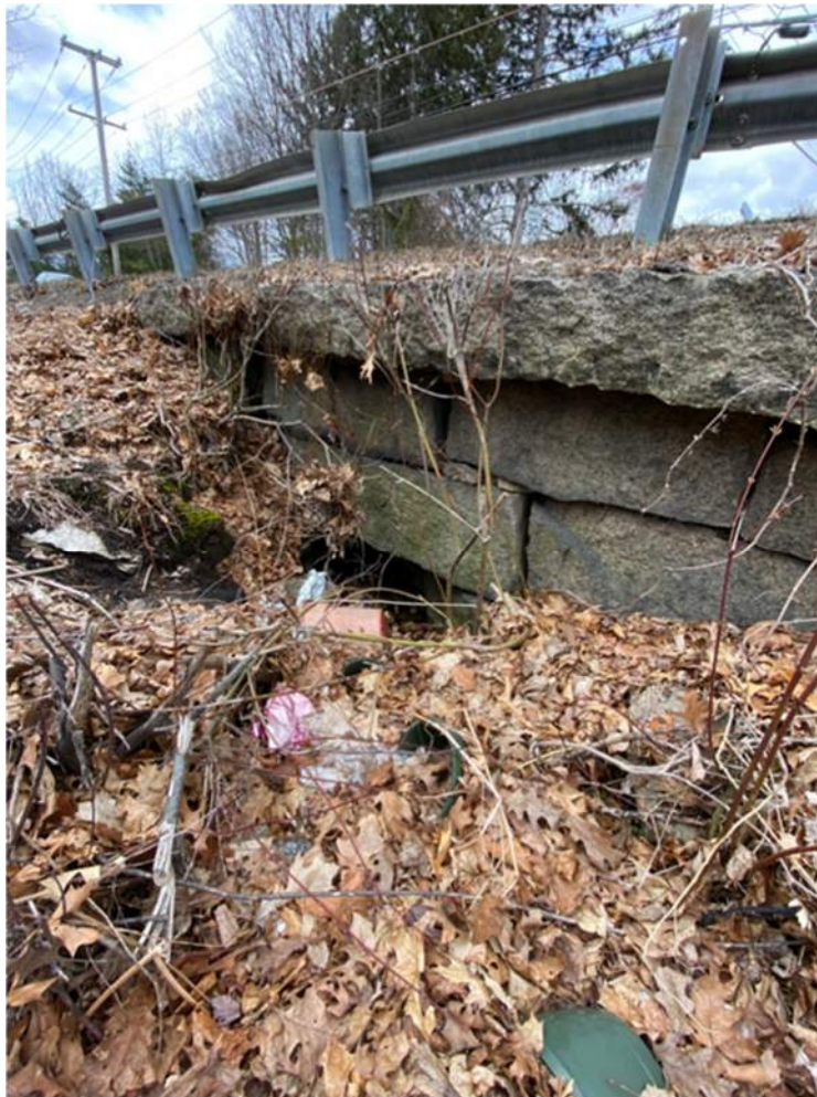
Photo 15 Fountain Street culvert, upstream headwall
